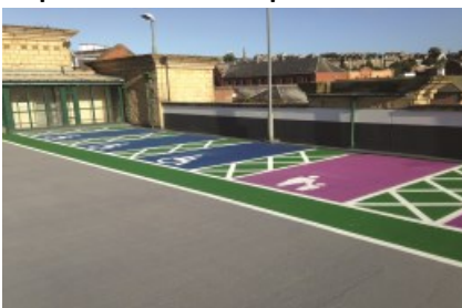
Exposed Deck & Ramps
