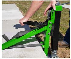
**Step 7.**After making sure the pins are in the jack foot and lifting loop and jack is plumb, start turning handle clockwise to start the lift.
